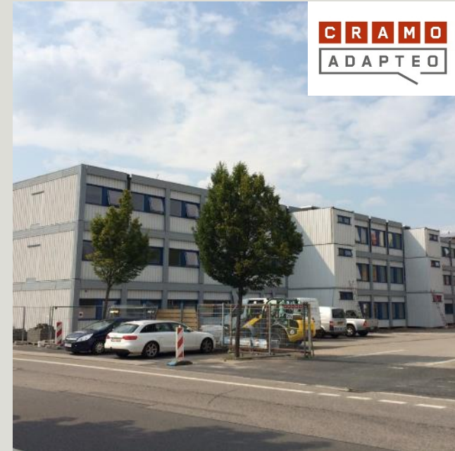
Temporary modular building in Germany 2015
